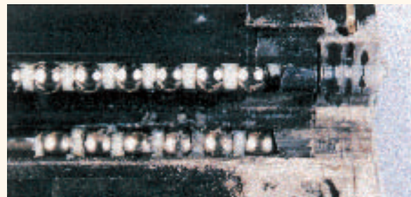
A large amount of foreign matter is present on the ball rolling surfaces.
